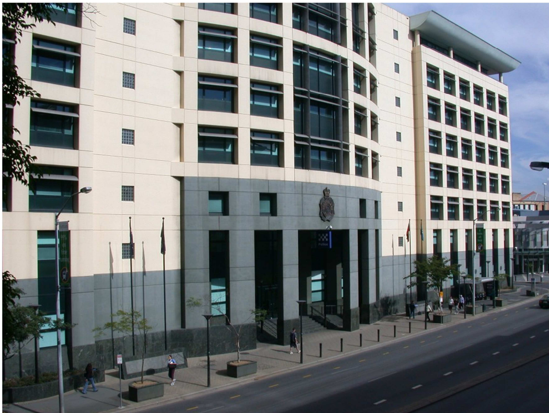
Queensland Police Headquarters, 200 Roma Street, Brisbane
